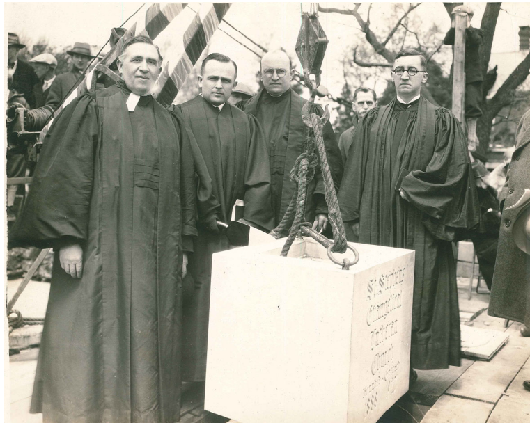
The cornerstone for the Broom Street building is laid during a ceremony on August 24, 1927.
